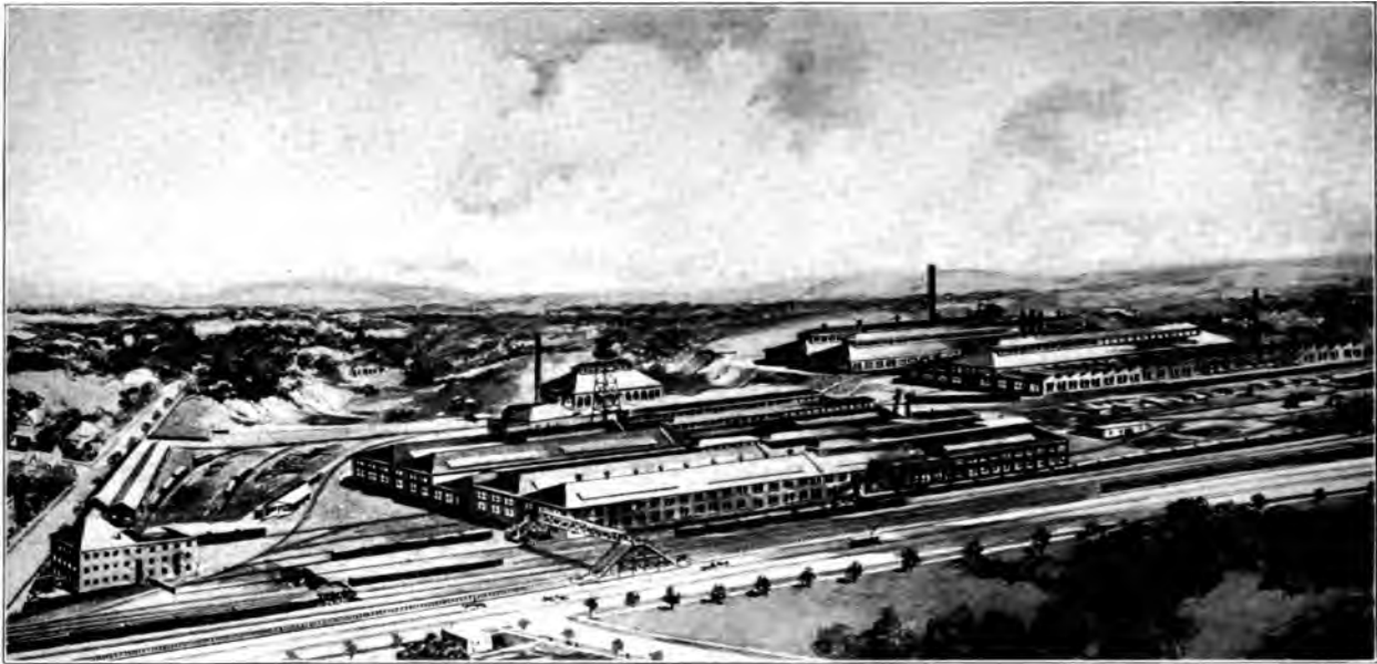
General Office and Works of The Union Switch & Signal Co. at Swissvale, Pa.
